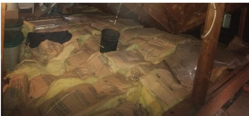
Kraft/Paper side is wrong side up and very uneven install with gaps
