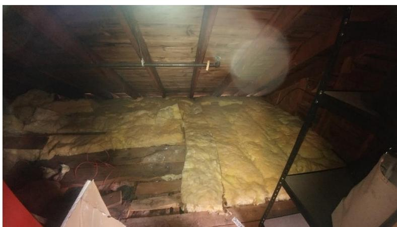
Gaps between rolls of fiberglass batt
