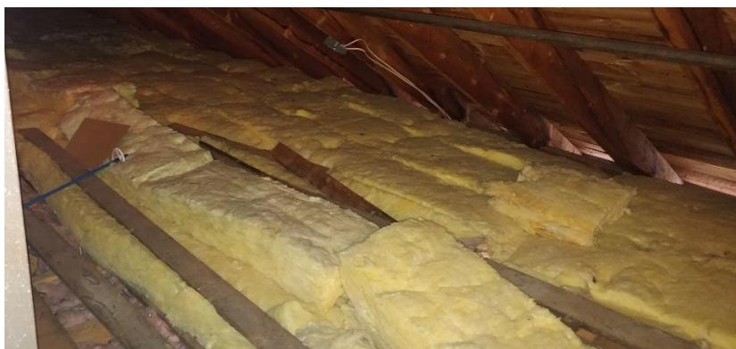
Uneven Install and Gaps. Insulation over exterior wall plate?
